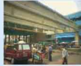
PC I-girder, 1 Spans 22 Nos, L 40m - H 1,85m ( under construction )
