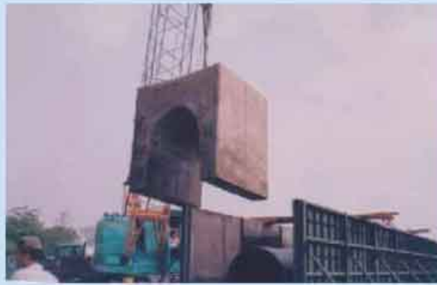
Retained Earth Pasupati Bridge - Bandung Supply concrete block system machine
