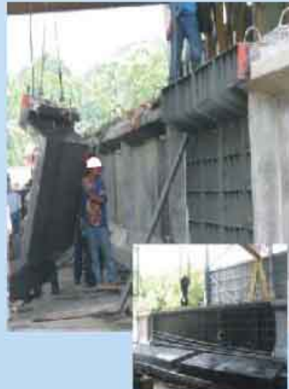
Surabaya - Madura Bridge, East Java Segmental PC I-girder, L40m-H 2,1m
