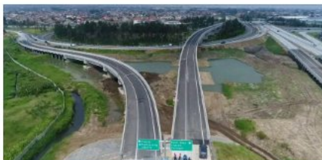
Proyek Jalan Tol Soreang – Pasir Koja
