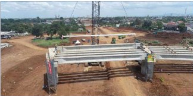
Girder Supply and Installation Depok Antasari Toll Road Package 1, Brigif Section
