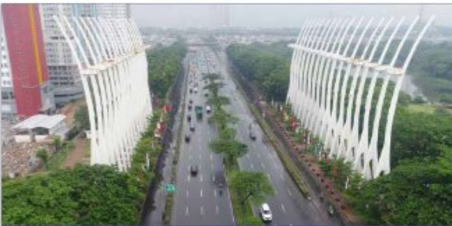
Kemayoran Toll Road Widening Project
