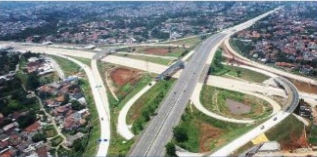
Depok – Antasari Toll Road Package 1 South
