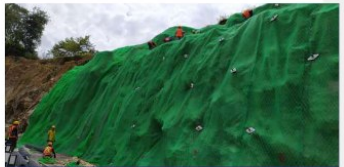
Rampa – Poriaha Mungkur Slope Stabilization (WINRIP)
