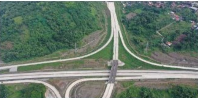
Cisumdawu Toll Road Project Section 3
