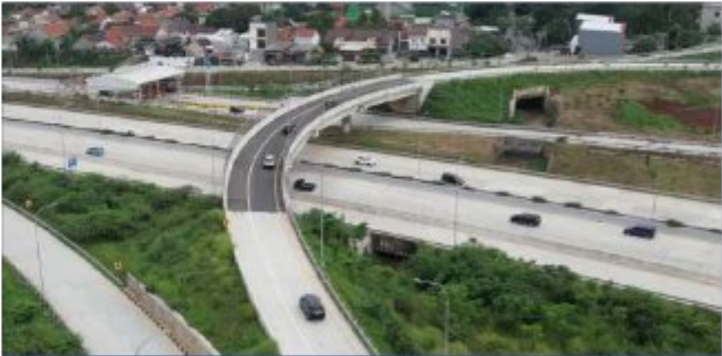
Krukut Bridge (Ramp 8) Section 1 South
