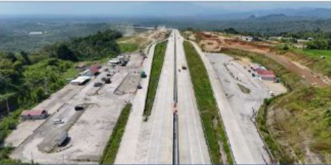
Rest Area Development Cisumdawu Toll Road
