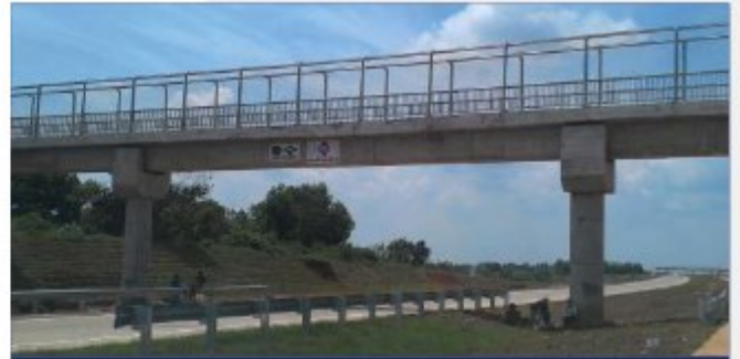
Cipali Toll Road Bridge Project
