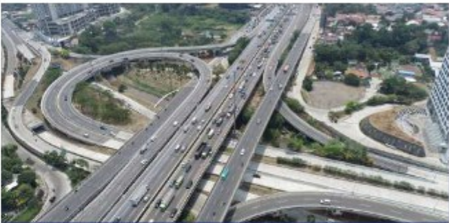
Depok – Antasari Toll Road Package 1 North
