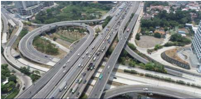
Depok – Antasari Toll Road Package 1 North
