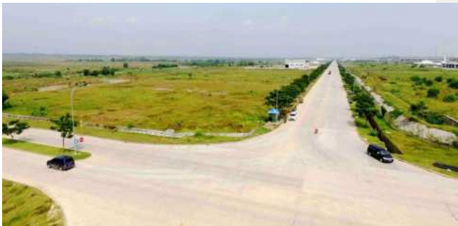
Deltamas Area Road & Drainage Project
