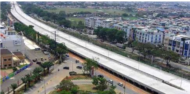
JORR W1 Toll Road Package 6 and 7
