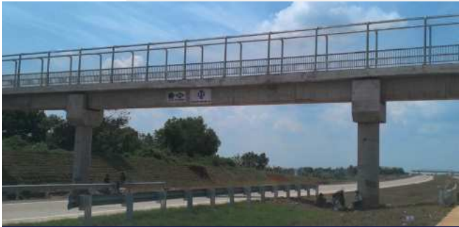
Cipali Toll Road Bridge Project
