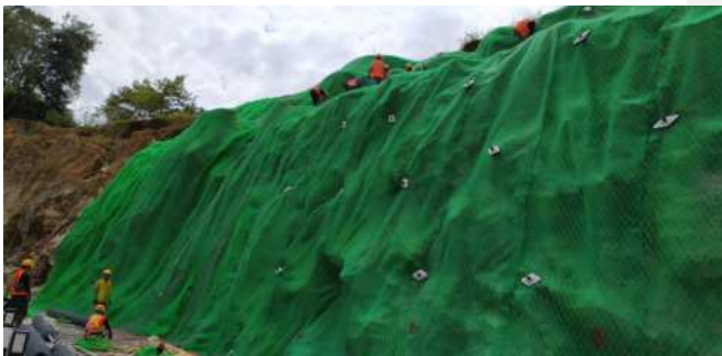
Rampa – Poriha Mungkur Slope Stabilization (WINRIP)
