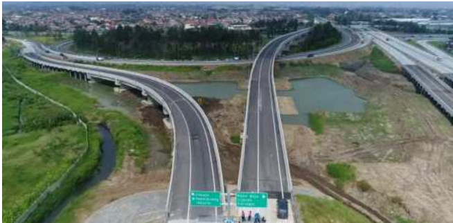
Soreang – Pasir Koja Toll Road Project
