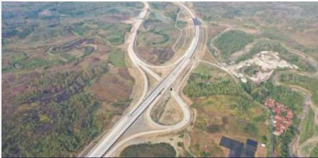
Cisumdawu Toll Road Project Section 6A
