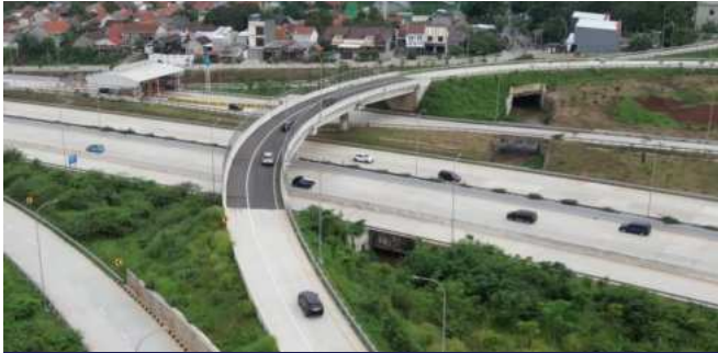
Krukut Bridge (Ramp 8) Section 1 South
