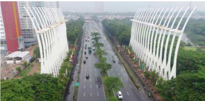
Kemayoran Toll Road Widening Project
