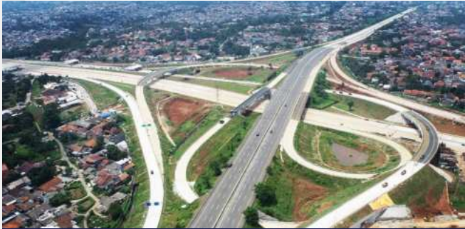
Depok – Antasari Toll Road Package 1 South
