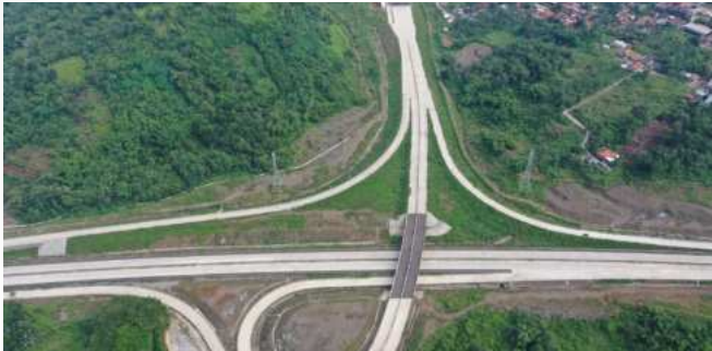
Cisumdawu Toll Road Project Section 3
