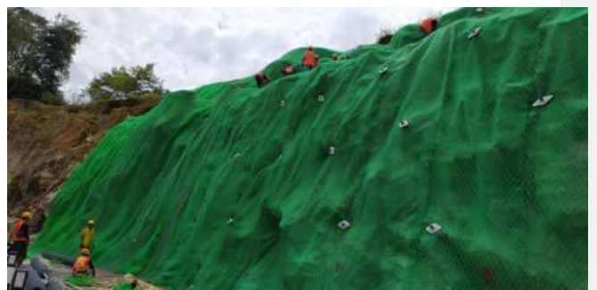
Proyek Stabilisasi Lereng Rampa – Poriaha Mungkur (WINRIP)
