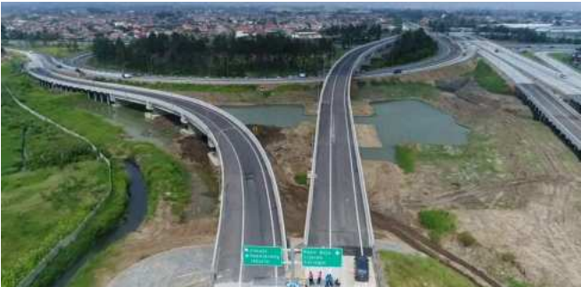
Proyek Jalan Tol Soreang – Pasir Koja
