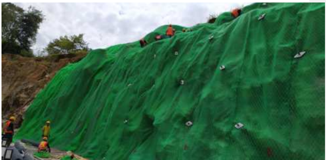
Rampa – Poriaha Mungkur Slope Stabilization (WINRIP)
