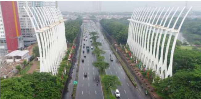
Kemayoran Toll Road Widening
