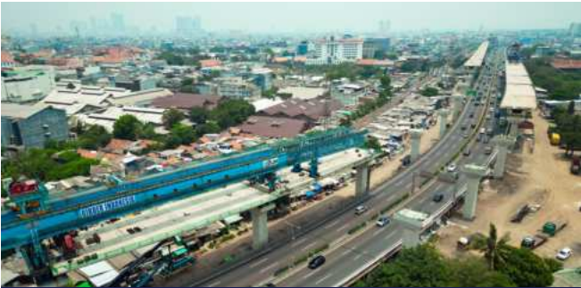
Ancol Timur – Pluit Toll Road (Elevated)
